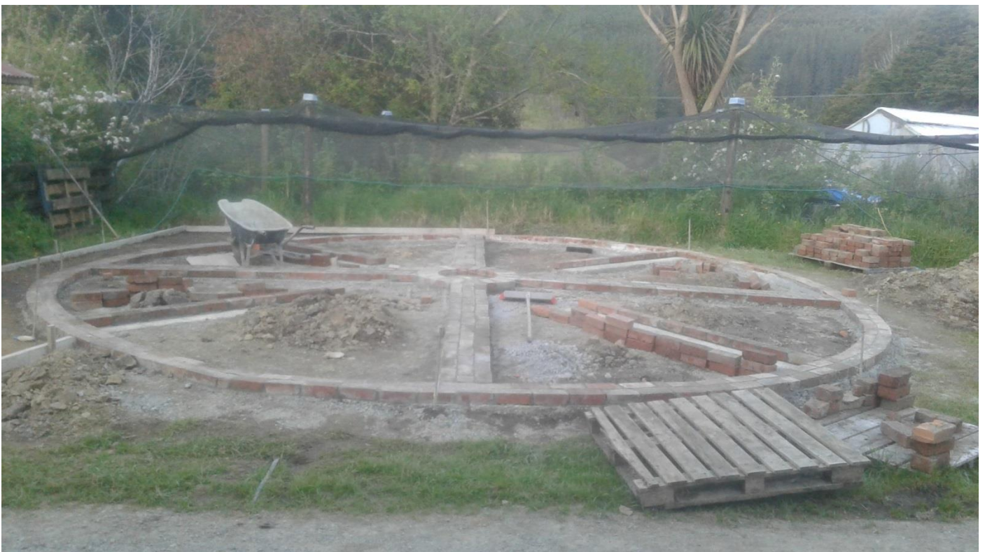
Bricks mortared on top of concrete
