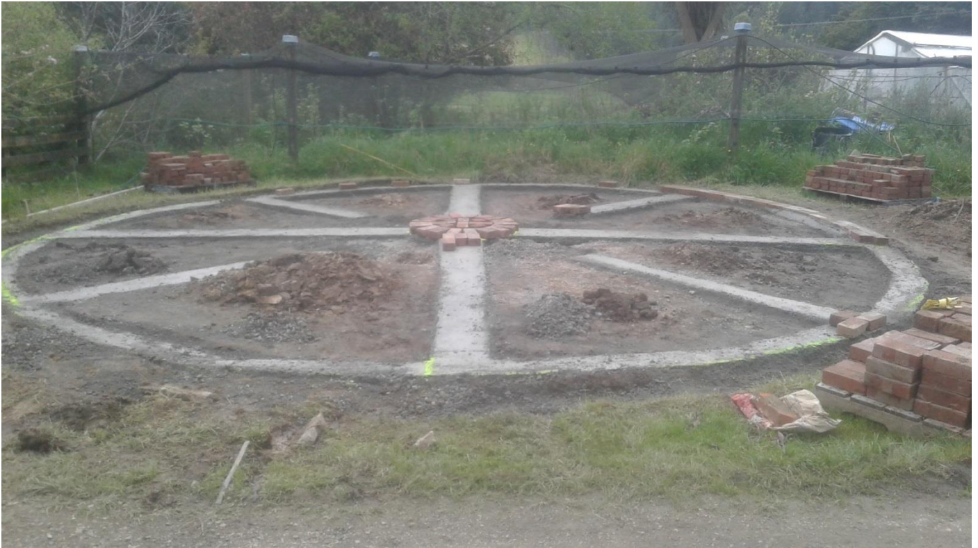
Concrete foundations in place
