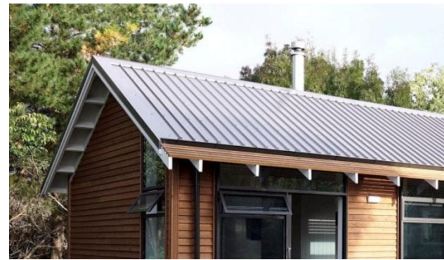
Figure 11: Slats on eaves – Greenhaven Smart Home
