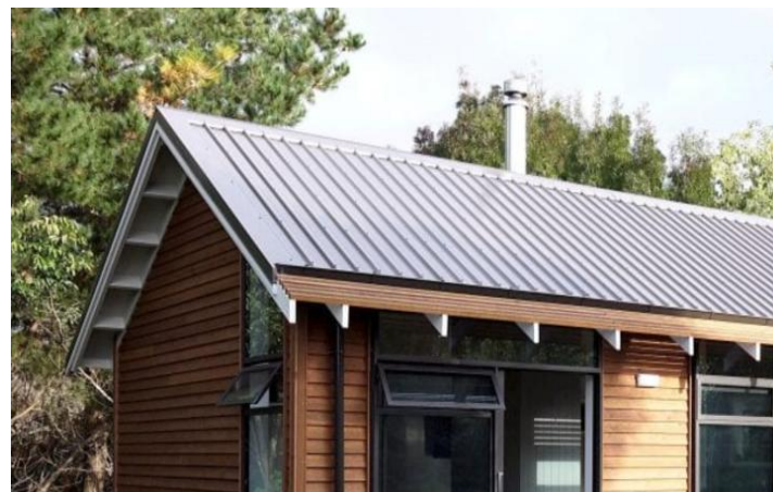
Figure 18 Slats on eaves – Greenhaven Smart Home
