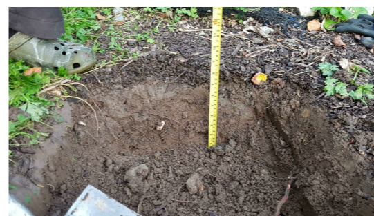
2. Measuring the hole 500-500mm x 150-200mm deep
