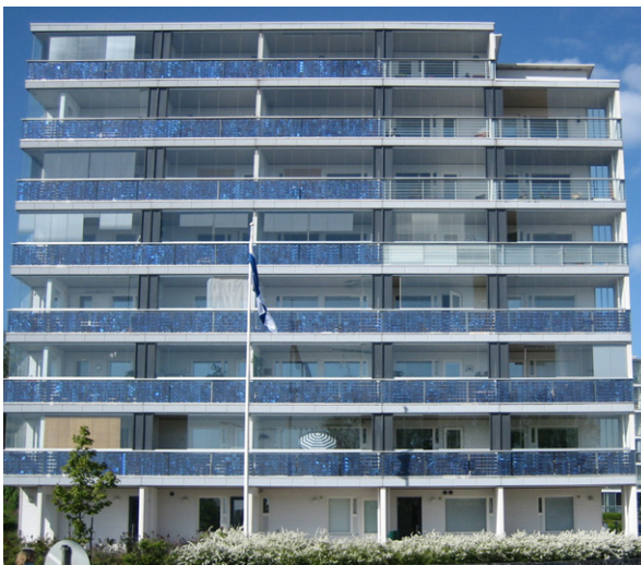
Figure 1 Solar panels, integrated in a block of flats in the Latokartano ecological housing area (Helsinki, Finland). https://upload.wikimedia.org/wikipedia/commons/6/66/Solar_panels_integrated_in_a_block_of_flats_in_Viikki_Helsinki_Finland.jpg Credit: Pöllö.
