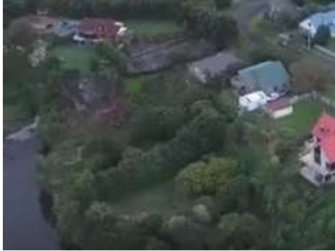
Figure 9: This more recent drone photo shows the new structure on 40 Kawei Rd, before more vegetation was cleared.
